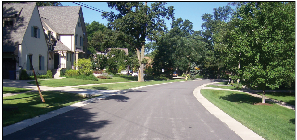
The Village's new road standard incorporates concrete shoulders, which help to extend the life of the pavement and reduce maintenance costs.
