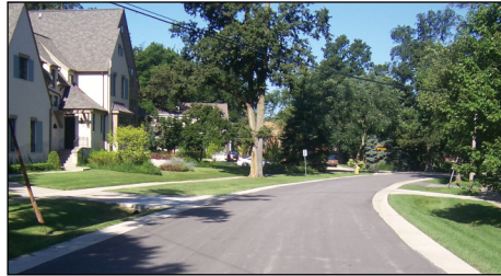
The Road Program will incorporate the Village's new road standard, which uses concrete shoulders.
