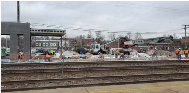
Installation of platform with snowmelt
