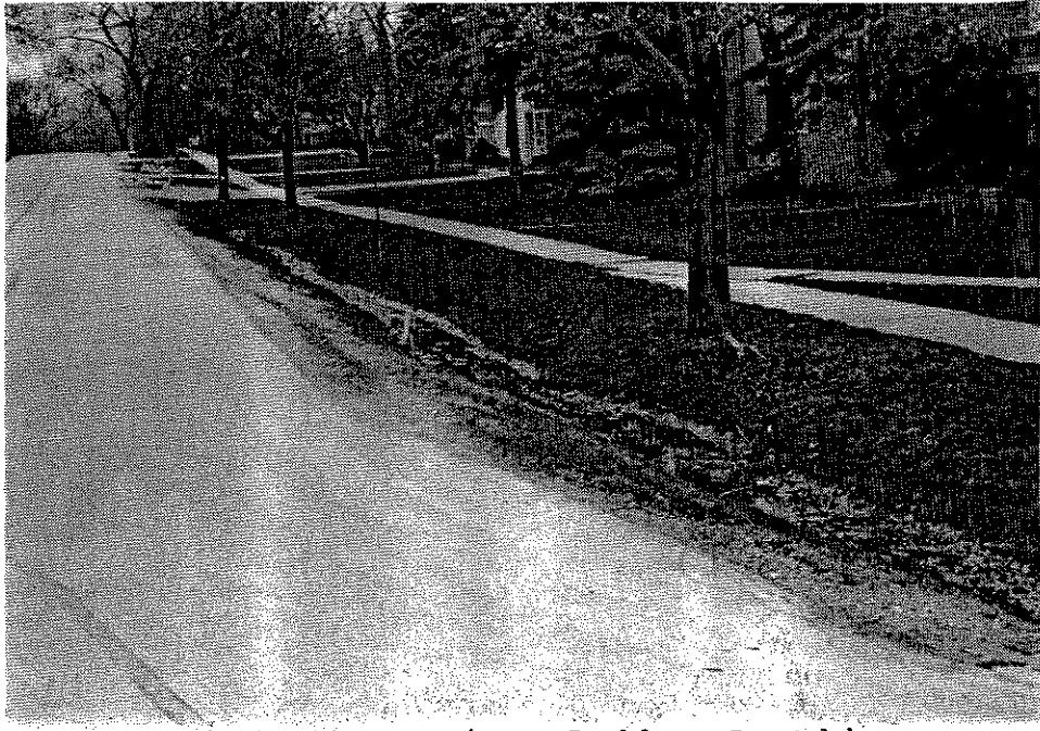
Figure 14. - Drainage Problems Caused by Uncleared Ditch
