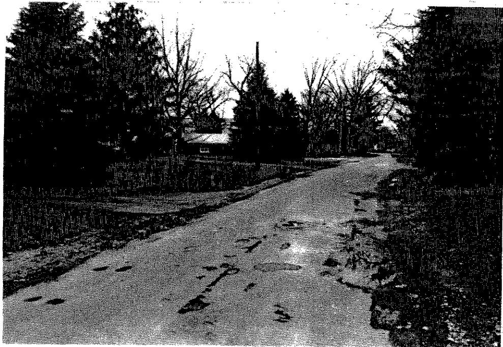
Figure 13. - Drainage Problems on Roads
